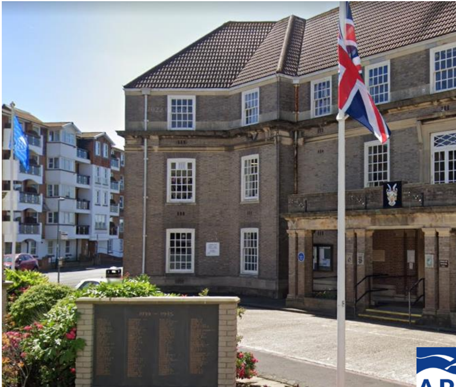
Photos of site
